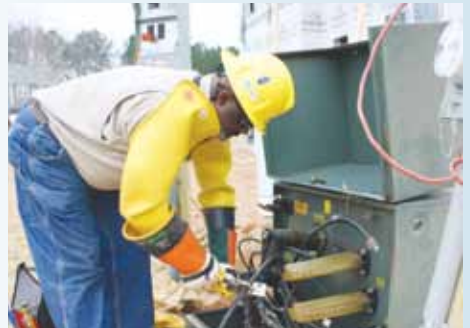
Equipment Operator Willie Champion uses protective safety gear as he works on an underground transformer.
